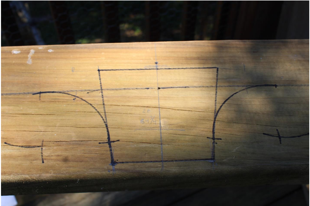
The keystone area was marked off in the exact center
