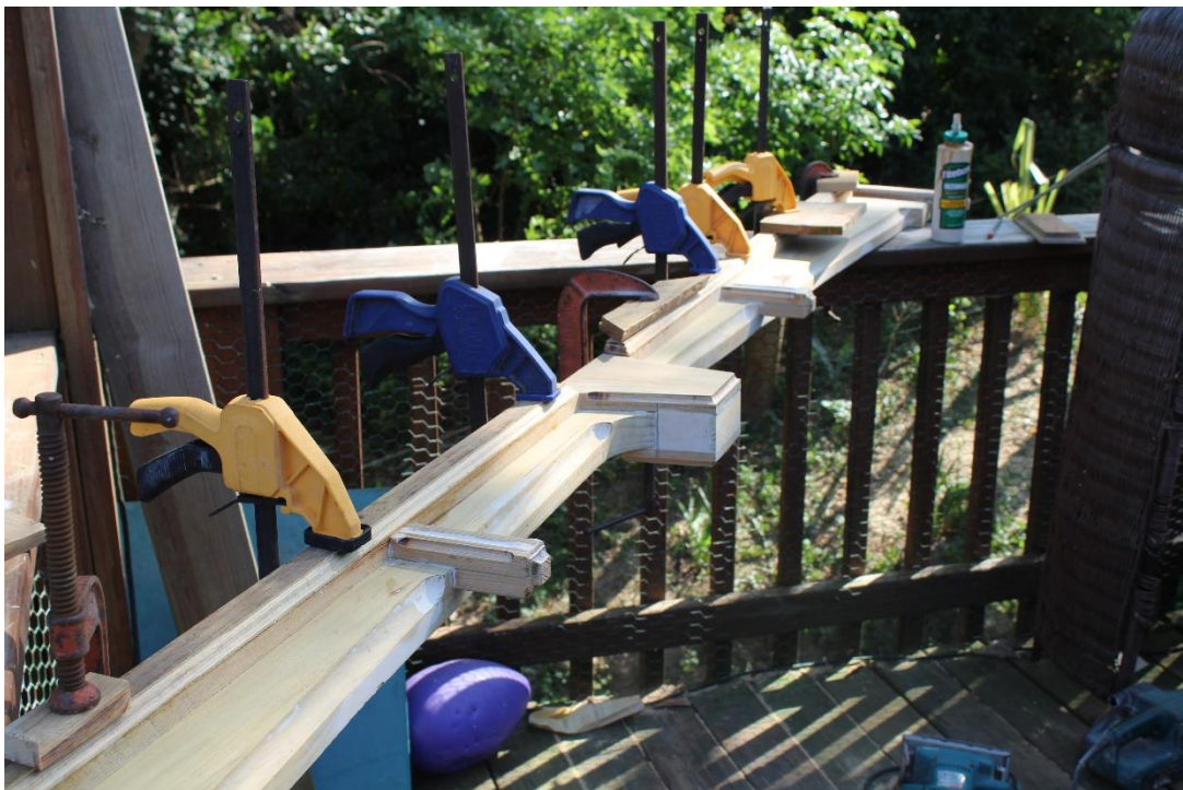
Detail routing complete and upper moulding in place
