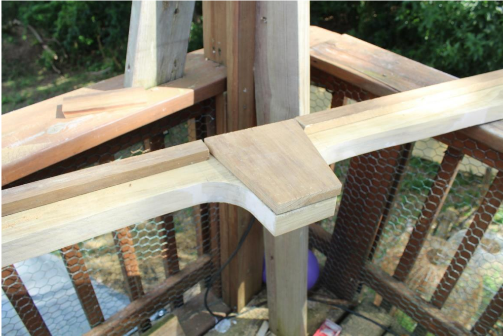
The keystone face and upper moulding base cut to size
