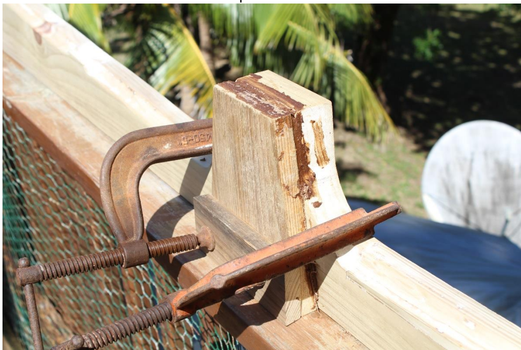
Glueing Keystone front face. Back face was the same
