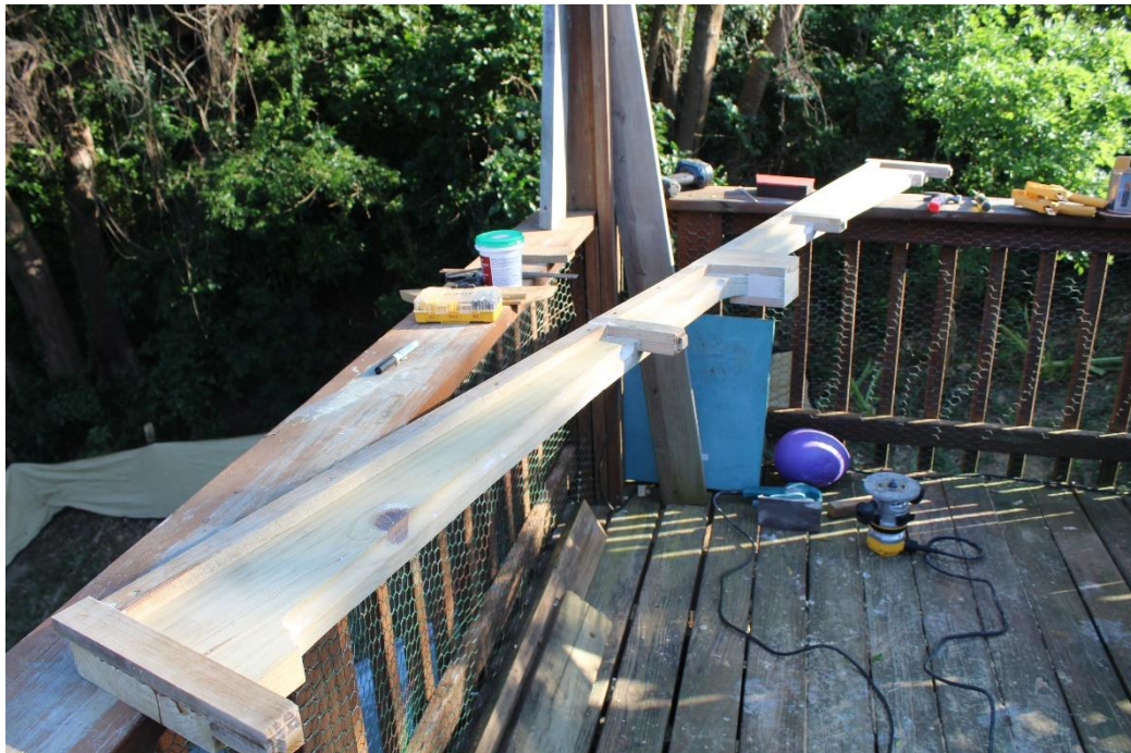
Outer spindles and upper moulding base glued in place.
