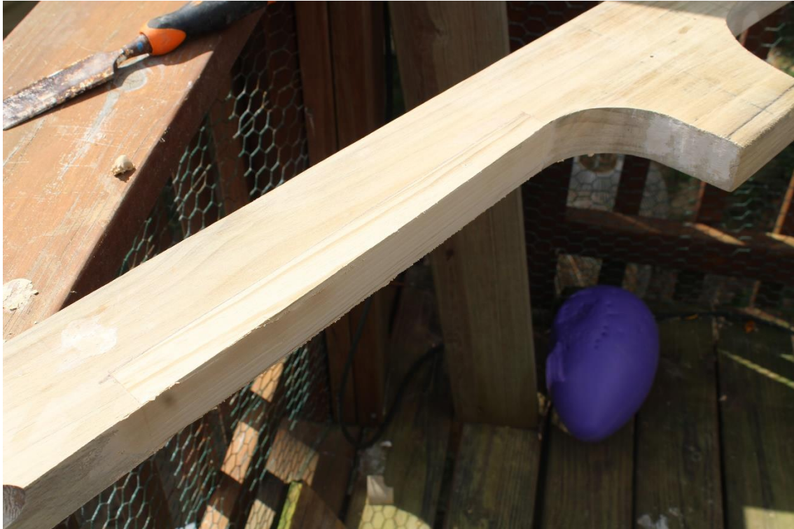
Finished repair came out well
