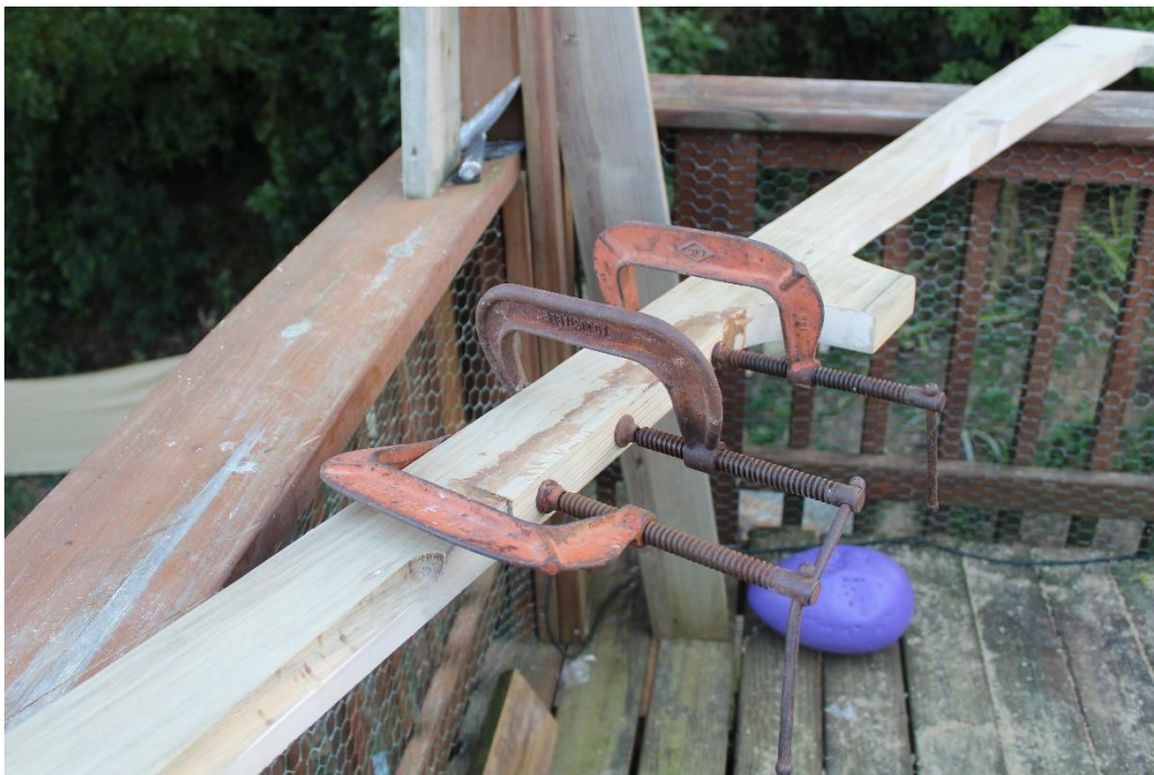
Disaster struck and a whole day was lost when the pin guide on the deep cove router bit came off and deeply gouged the wood. Had to insert a 2"x 2"x 12" piece of wood and re-contour the arch.
